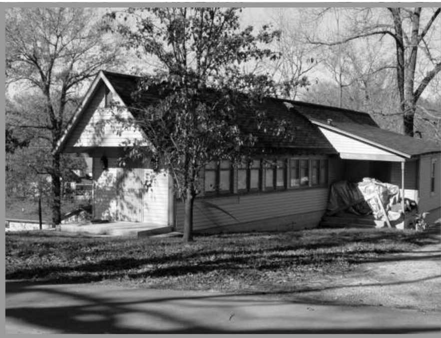
This house, in Cadiz, KY, was initially a Cadiz RR coach. Engineer, Dickie Mitchell, got the retired coach in 1938 and with the aid of 150' of temporary track and a Cadiz locomotive put the car in position, removed the wheels and set about completing the home. digital image by Chuck
